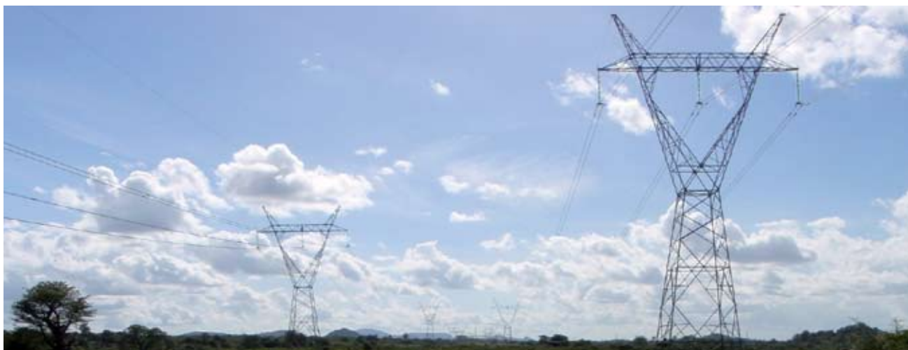
Cahora Bassa power lines run right past the project.
